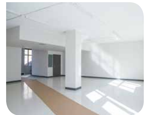
The just completed Tenants Association room, complete with a full kitchen.
